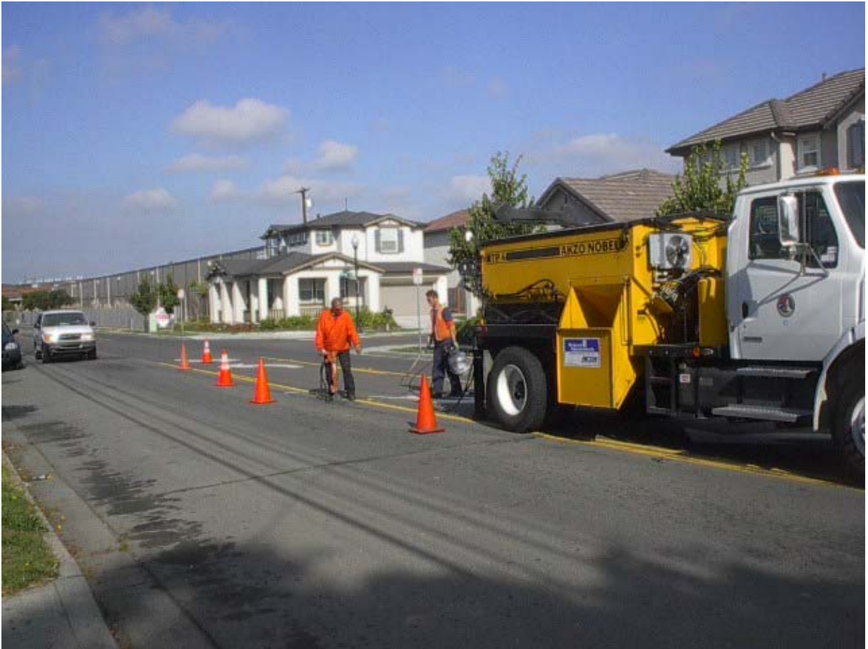
Pothole Patching (Local Streets and Road funds)
