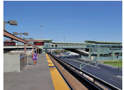
Rendering showing link from BART's Coliseum station to the Oakland Airport Connector.
